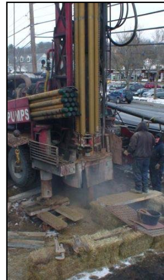
Geothermal well drilling in process. Photo courtesy of Nexamp.
